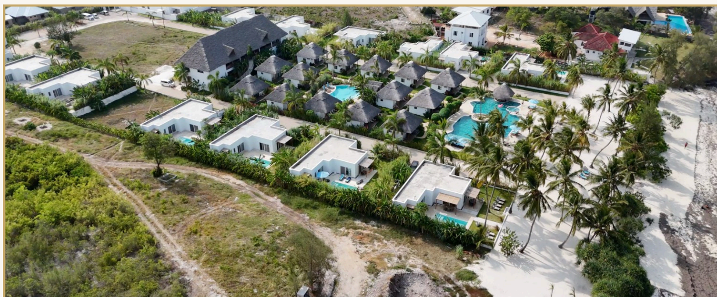
Photo of the overall compound
