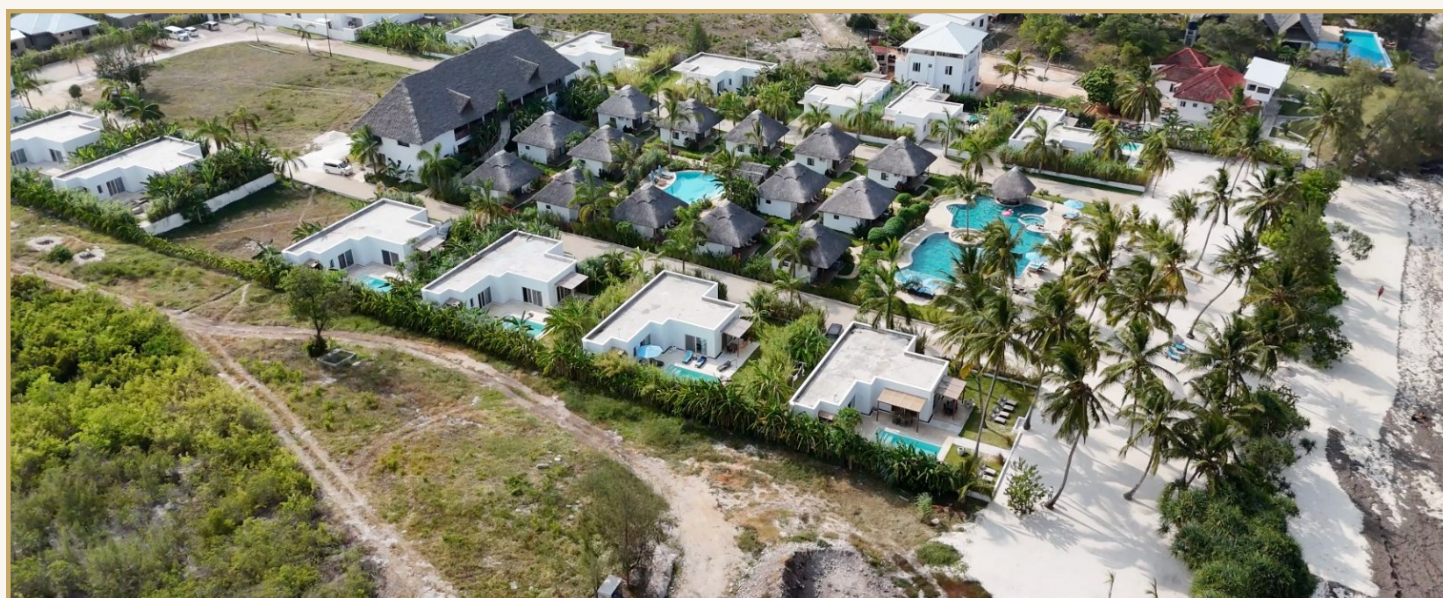
Photo of the overall compound
